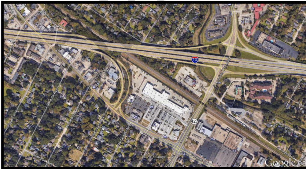
Figure 2.2 Acadian Perkins Interchange Source: Google Earth
